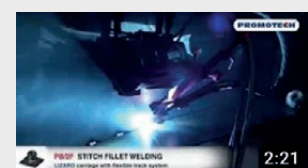
Horizontal Fillet Welds | Welding in PB / 2F position
